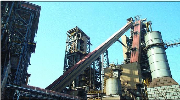
● **Figure 6** Largest inclined bucket conveyor for hot material with inertisation
