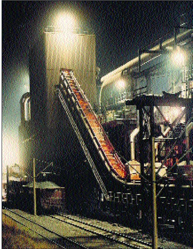
● Figure 3 Example of hot material transport system in the 1960s
