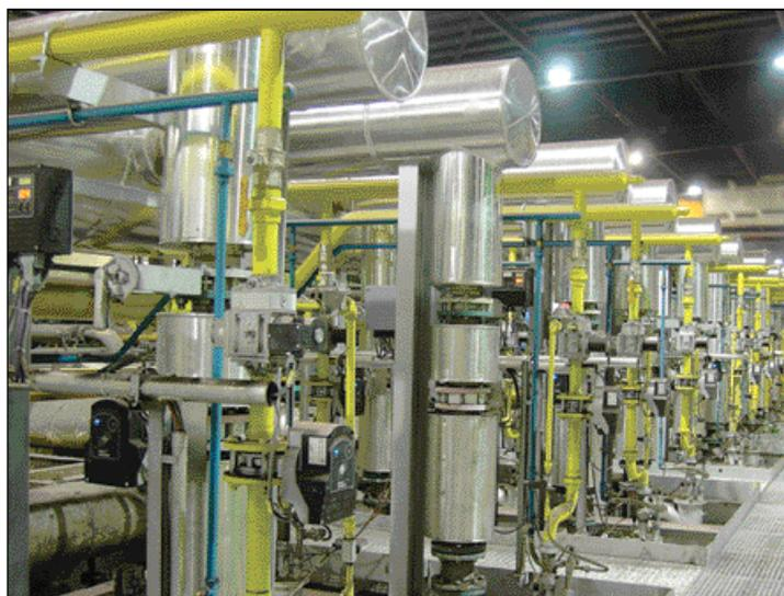
● **Figure 8** Heating system of the ceiling burners
