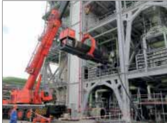
Fig 4 Removal and installation of bundles
