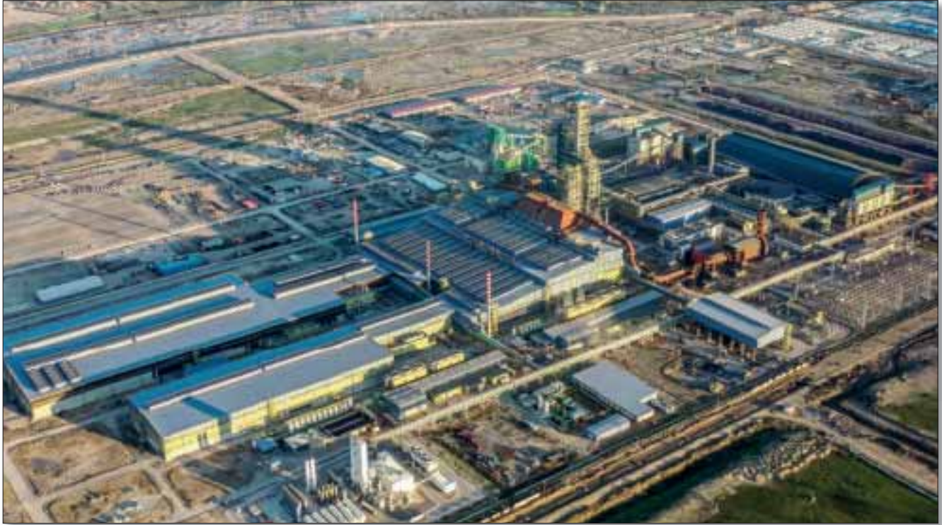
Fig 3 DRI plant of Algerian Qatari Steel (AQS), supplied by MIDREX with Paul Wurth
