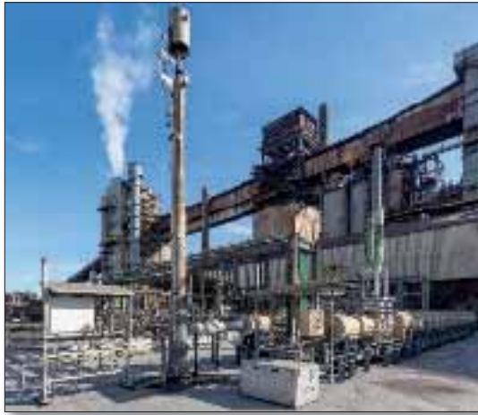
📍 Fig 2 Pilot plant for syngas generation at ROGESA
