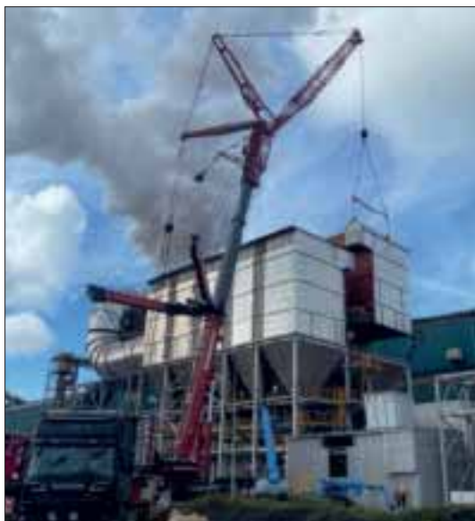
📍 Fig 6 Installation of the final module
