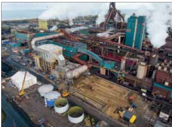
📍 Fig 7 Completed installation
