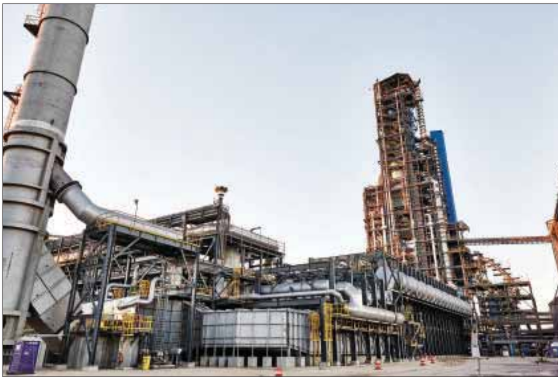
Fig 3 Corpus Christi HBI plant
