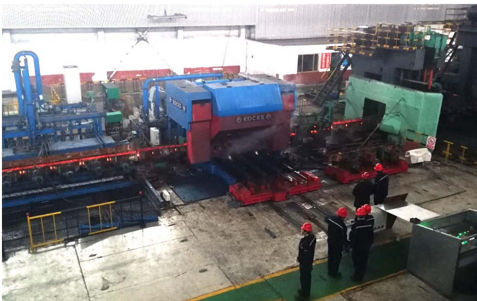
Commissioning of KOCKS 3-roll RSB® 5.0 in Weifang
