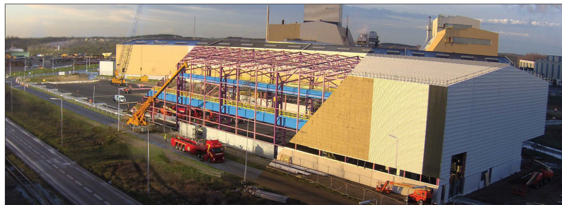
Fig 1 Phase three of the LA warehouse under construction
