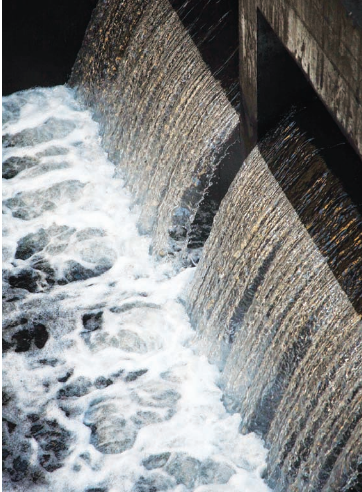
Ⓐ Fig.3 Decanting basin outlet
