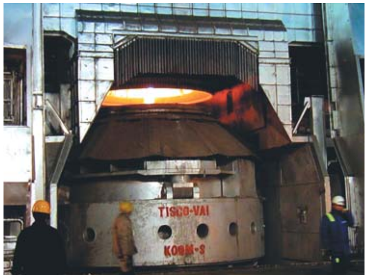
▲ Fig.3 Preheating of the K-OBM-S converter
