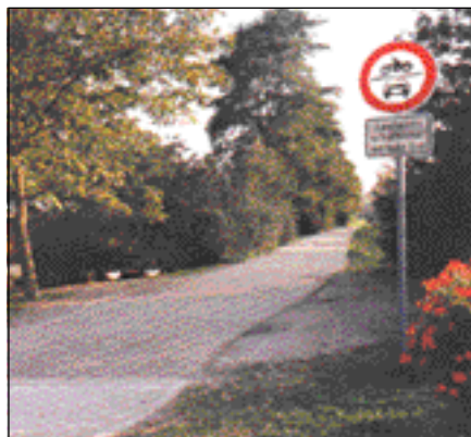
● Figure 7 Cartway in Black Forest made of EAF and LF slag
