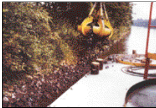
● Figure 6 Bank reinforcement at the river Rhine
