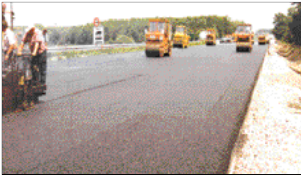
● Figure 5 Motorway in southwest Germany made of BSW slag
