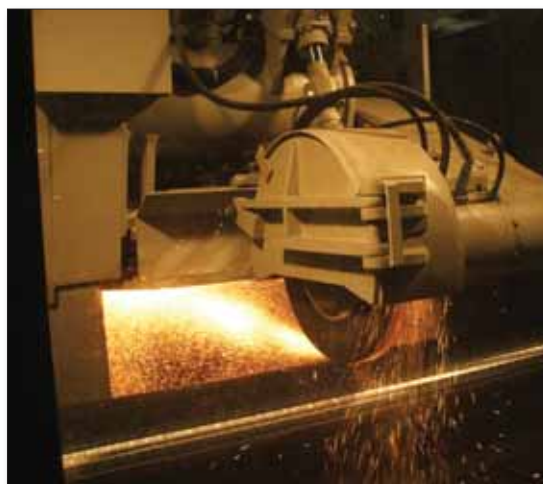
Ⓐ Fig 7 Grinding head in operation
