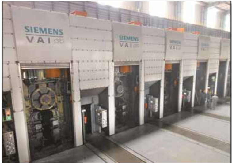
Fig 2d The completed cold mill
