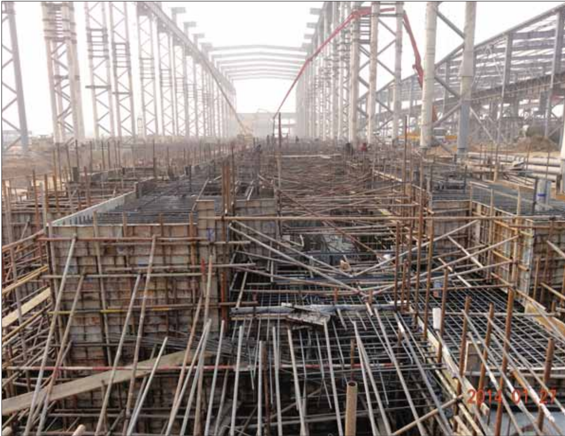
🕒 Fig 2a Construction activities in the cold mill complex area
