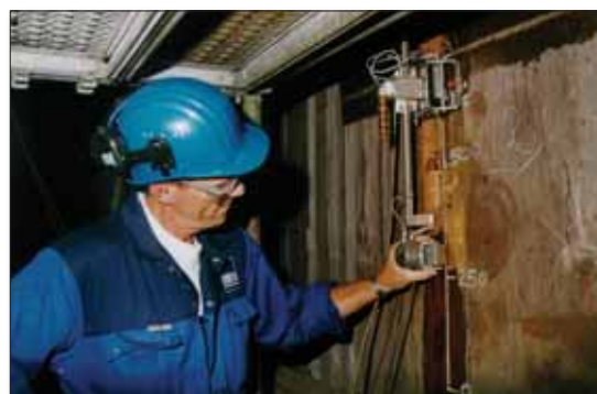
Ⓐ Fig 3 Non-destructive testing of a steel shell
