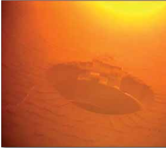
Fig 5 Endoscopic condition monitoring
