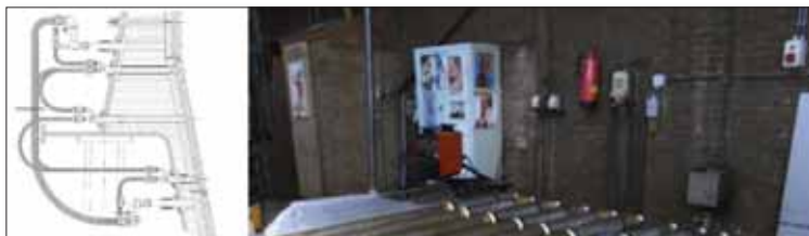
Ⓐ Fig 10 Installation of additional cooling capacity from outside the furnace
