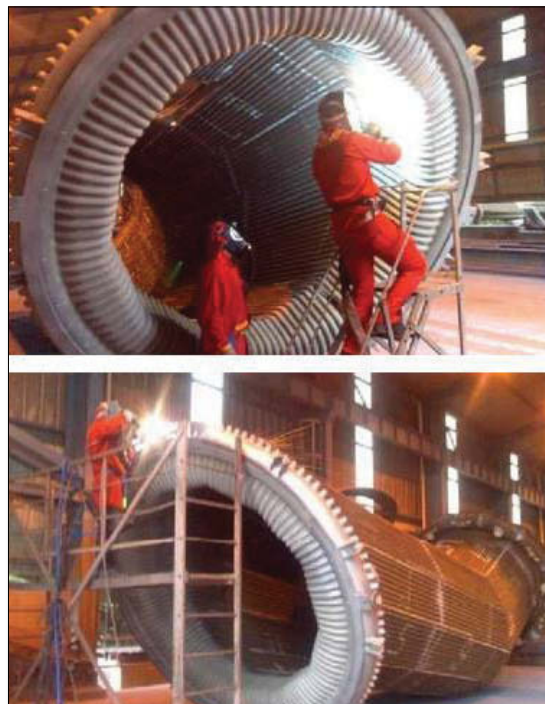
📌 Fig 13 Spraying of EAF gas ducting
