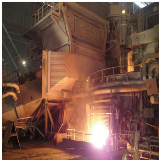
Fig 5 110t COSS system operating in North Europe
