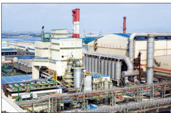
Fig 6 Primus dust recycling plant
