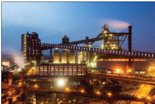
Fig 4 BF '1', 2.5Mt/yr ironmaking plant of TATA Steel Ltd, Jamshedpur, India
