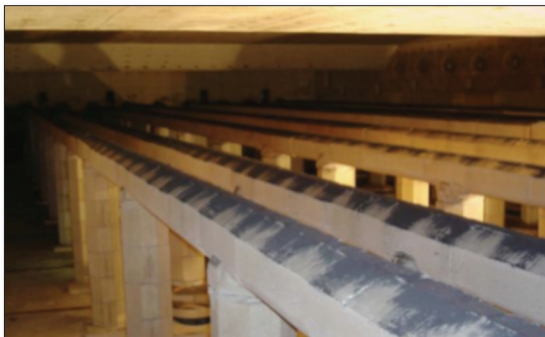
Fig 3 iRecovery@skid system for a 200t/h walking beam furnace
